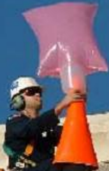
Unit Valve/Blow Down Valve Leakage
